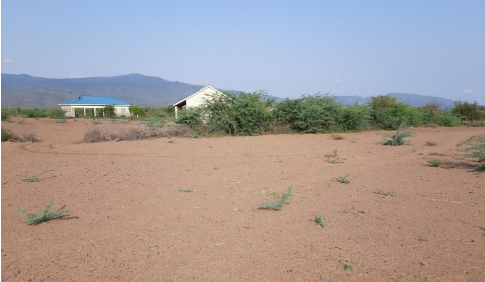
Naremiato primary pit latrines Construction of 2 blocks of Pit latrines GPS: N 4 5'35'' E 34 32' 54''
