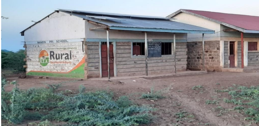
Namon primary pit latrines sub-project construction of 3 blocks of pit latrines GPS: (e) 442781 (n) 707821
